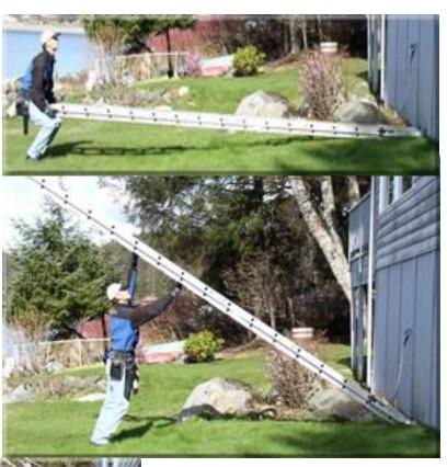
**Second** - lift ladder's top while pushing forward to maintain pressure against building's wall. \*Don't perform ladder work if you are not mentally or physically capable of safely accomplishing the work. \*Lift with your legs, not your back.
